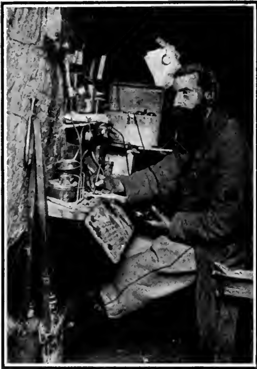
IN A FRENCH TRENCH. -A Telephone Operator at work.
